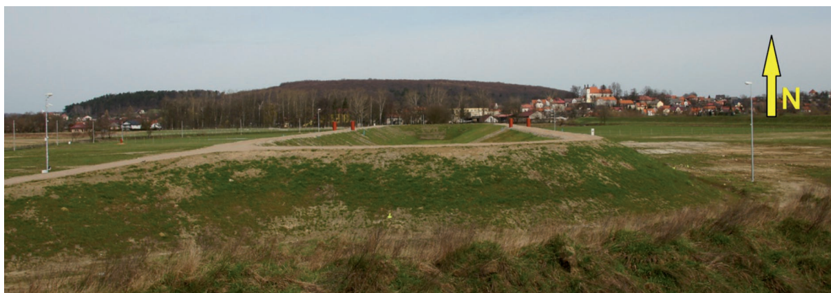
Fig. 1. Photograph of the experimental embankment
